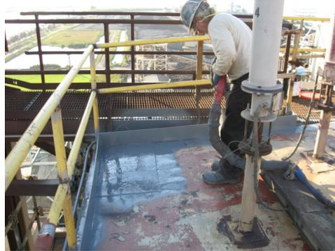
Industrial Maintenance Group applied approximately 80 mils of high heat resistant coatings to the above pictured precipitator units within a coal fired power plant located in central Florida. A non-slip surface was provided for a safe walking surface on each unit.
